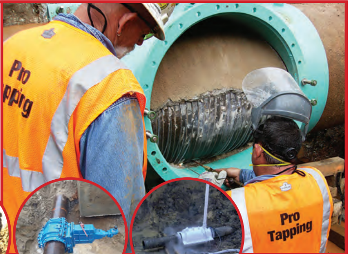
30" X 24" Wet Tap on PCCP Water Line
