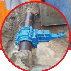
16" Horizontal Valve Insertion on DI Water Line
