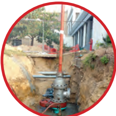
10" Line Stop on CI Water Line
