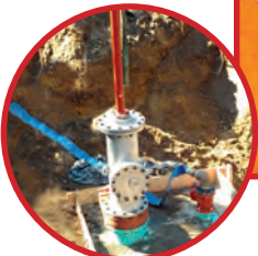
16" Line Stop on CI Water Line
